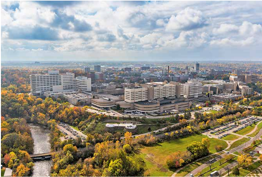
Snimka iz zraka: Michigan Hospital Michigan Medicine – University Slika prenesena sa: https://www.freep.com/story/news/education/2020/05/05/michigan-medicine-furlough-workers-construction-hospital/3083978001/
